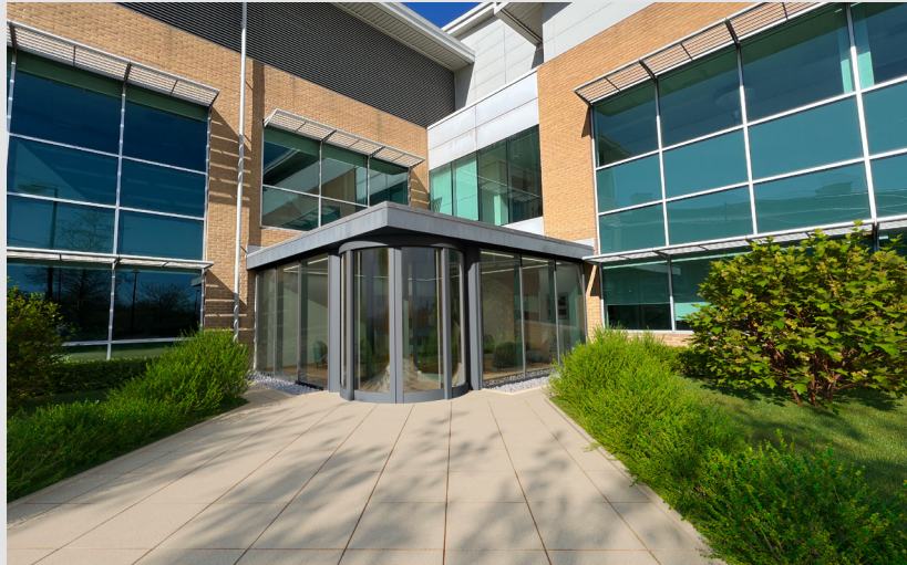
EXTERNAL FRONT ENTRANCE
