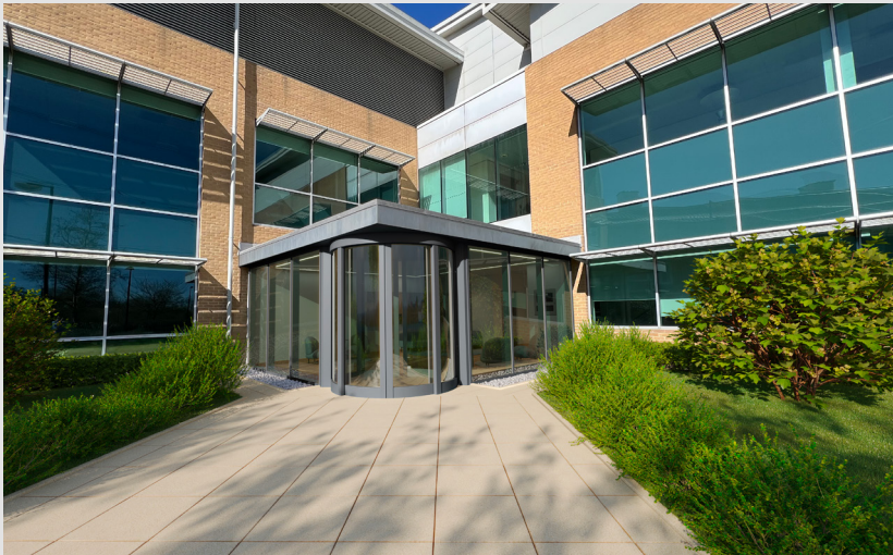
EXTERNAL FRONT ENTRANCE
